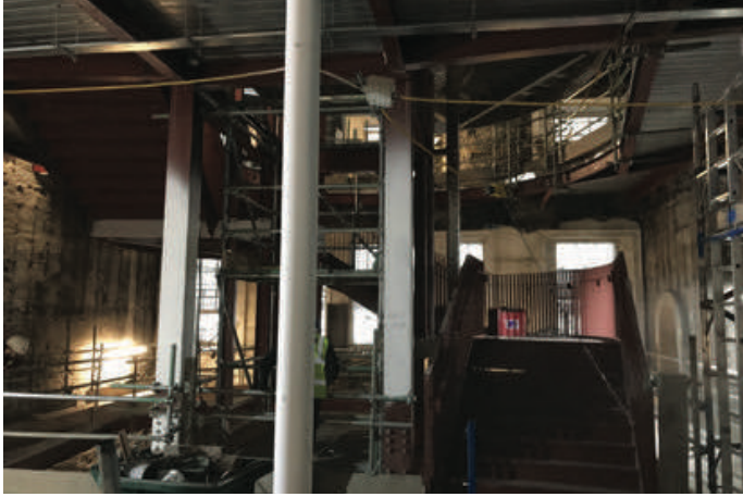
The main staircase was recently installed.
